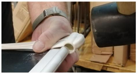
Using two people hold the canopy sheet in the groove and **GENTLY** tap the end of the bracket. Until the metal front bar locates into the bracket
