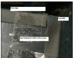
A good tip here is to tape the rubber seals into place with the long edge seals going to the end of the sheet and the short edges going between the rubbers on the long sides
