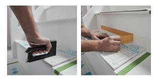
**3. Attaching the stair runner** Start at the top of the stairs, just underneath the bullnose. Then work your way down the stairs, securing the runner under the bullnose, at the edges and in the corners with an industrial stapler. Get a tight fit with a bolster chisel.
