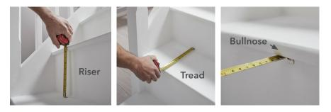
**2. Preparing the stairs** Mark each riser and tread with the painters tape to show where the runner should go. Then measure and cut the carpet underlay--- 20mm narrower (remember you only need padding for the tread) and attach with a staple gun. Add carpet adhesive tape to the riser.
